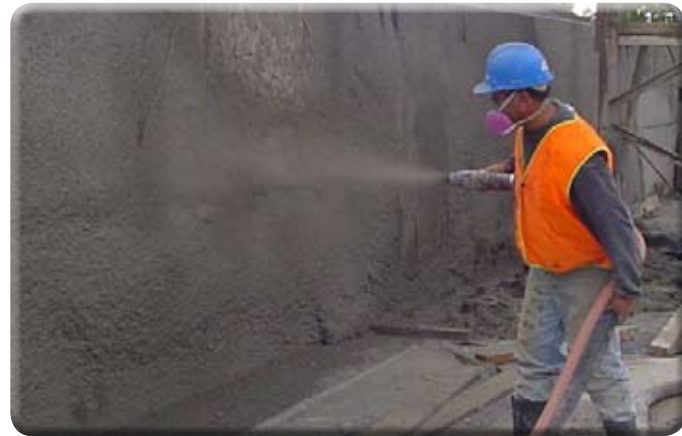
Figure 3. In place shotcrete performance depends on the operators skill.
