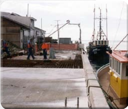
Figure 1. Microsilica 600 was used on the Motueka Wharf to give a 50 year life design
