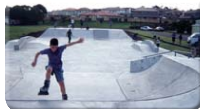
Figure 1. Microsilica 600 was used for the Titirangi Skate Park for ease of placing and superior abrasion resistance.
