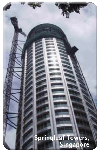
Figure 6. MS600 was used in concrete for high strength columns, reducing their size and giving increased usable area.
